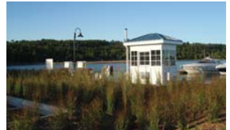
The newly rebuilt public facilities at Wisconsin's Egg Harbor Marina include "the most adorable fuel dock" on the Door Peninsula.
